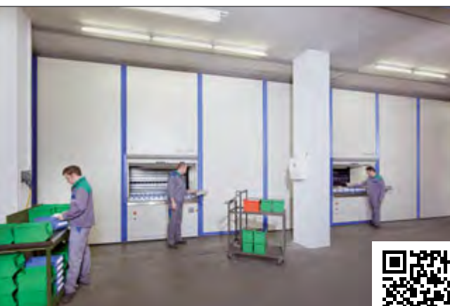
Two Hänel Multi-Space® units each 9.57 m wide constitute the central store for the production hall
